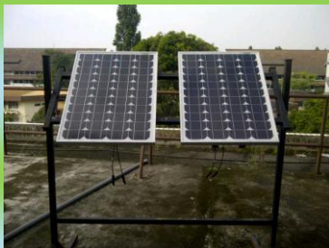
Figure 1. Installation of PV panels outdoor
