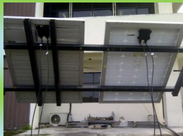
Figure 2. Back part of PV panels. Left panel is equipped with Al containing PCM
