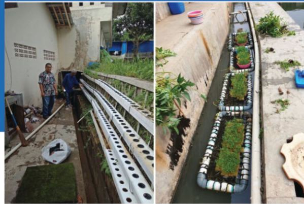
Figure 1. Constructing the Aquaponic System at Cinangsi District
