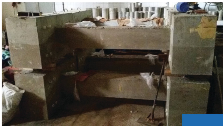
Figure 2. Structural elements made of green concrete with no OPC.
