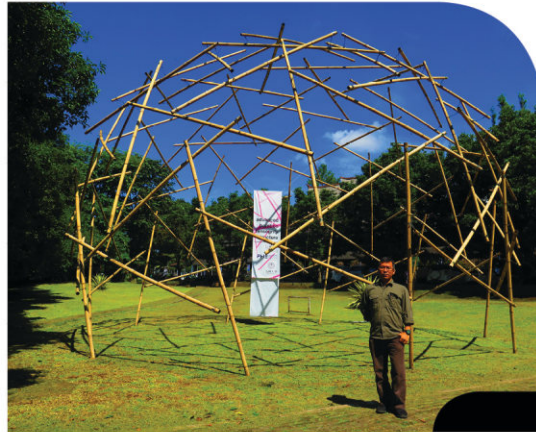
Figure 1. New structural system as combination between reciprocal frame and tensegrity called rection of reciprocal tensions.
