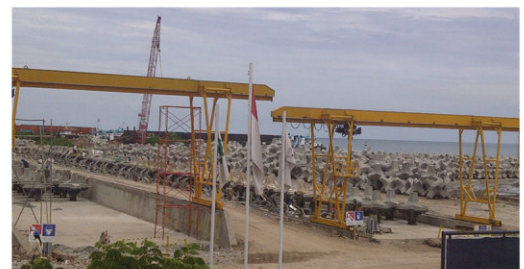
Figure 2. Application of Bamboo Matras and armor unit A-Jacks in Kali Baru Port, Jakarta (under construction).
