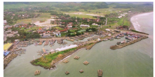
Figure 1. Application of Modified Caisson, Bamboo Matras and armor unit A-Jacks in Palabuhan Ratu Fishery Port: 1) Top left-right Cross Section and A-Jacks; 2) Middle left and right under construction; 3) Bottom right already in operation.
