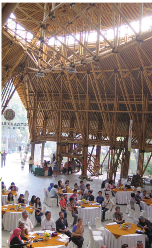
Figure 3. Great Hall Outward Bound Indonesia, huge bamboo structure with free span of 20 to 31 m, using more than 8000 bamboos.
